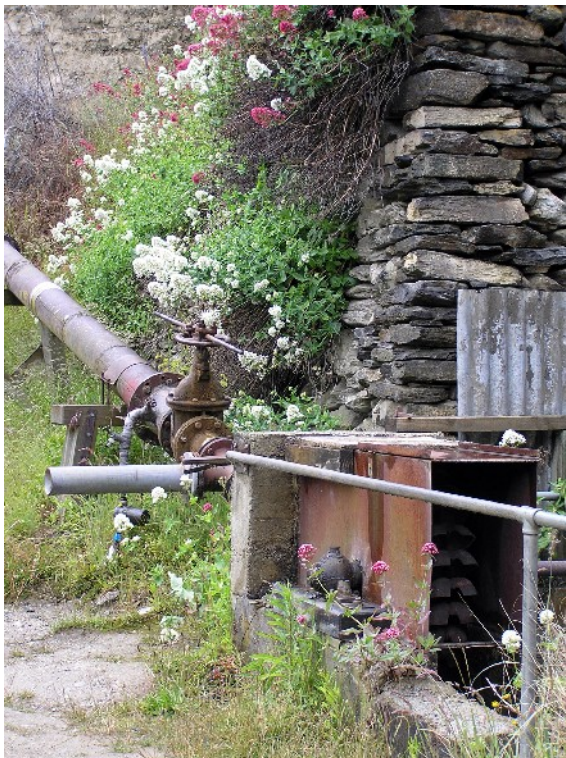
The pipe supplies water to a Pelton wheel. You can see its curved buckets in the rusty box
